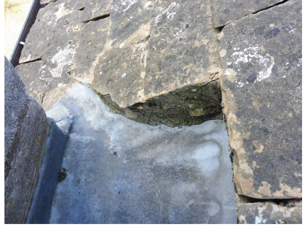
Nave/Lady Chapel and Tower lead lined gutter – Poorly detailed leadwork.
