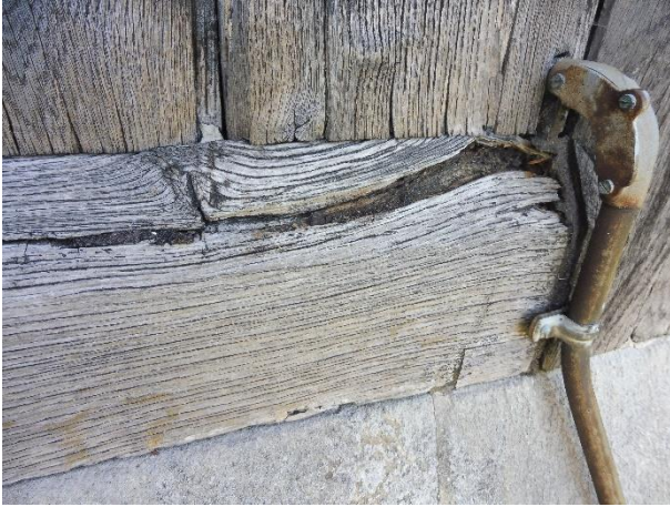
South Porch – Splits/shakes to timberwork.
