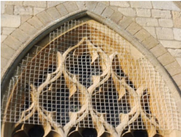
Chancel east gable - Rudimentary and inappropriate window guard.
