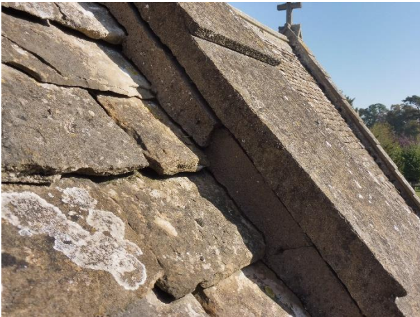
Nave east gable parapet – Cracked/damaged mortar fillet.
