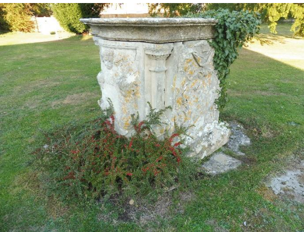
Churchyard monument – Displaced stonework and open joints.
