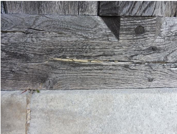
South Porch – Splits/shakes to timberwork filled with dense mortar.
