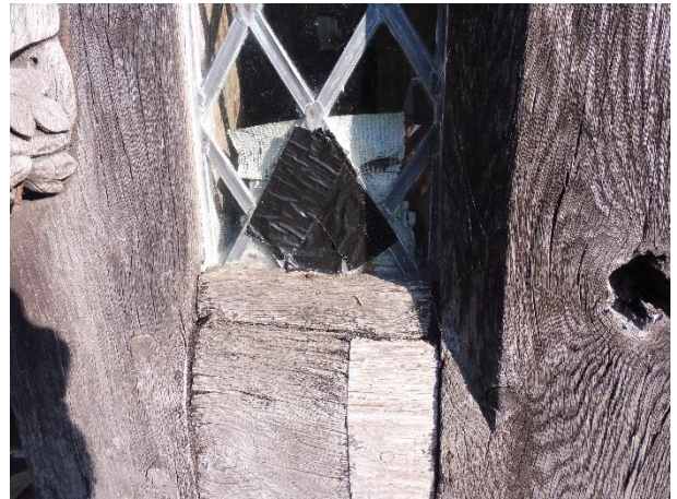
South Porch – Damaged glazing.
