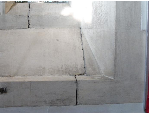
North Aisle – Movement through east window.
