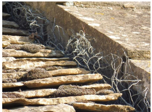
Lady Chapel, south – Wire mesh to lead lined secret gutter.
