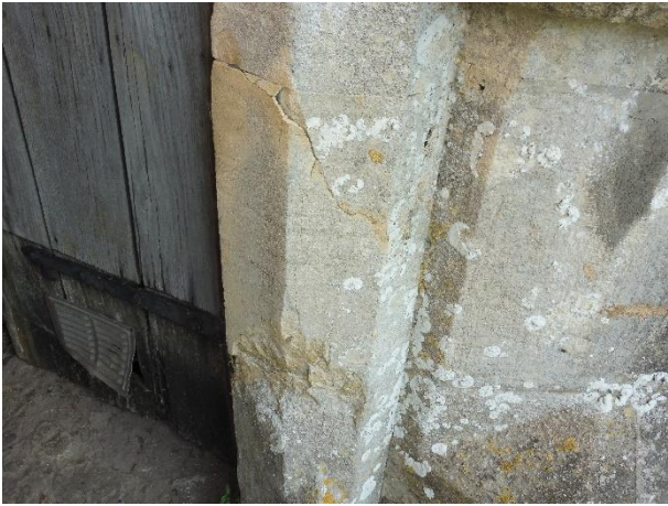
Turret staircase doorway – Fractured jamb.
