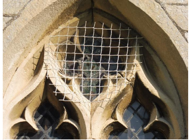
Lady Chapel – Rudimentary and inappropriate window guard.
