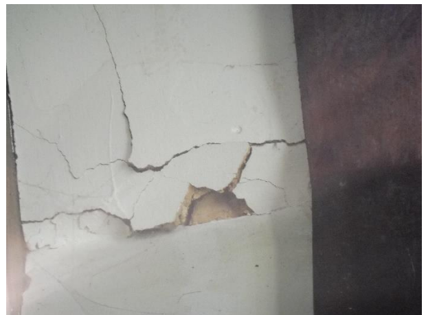
North Aisle – Damaged plaster.
