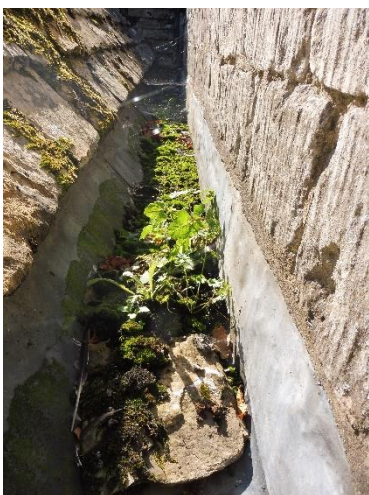
Vestry west lead lined box gutter – Vegetation, moss and debris.
