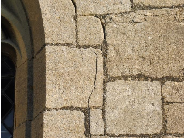
Lady Chapel, south window – Vertical movement and fracture to jamb.
