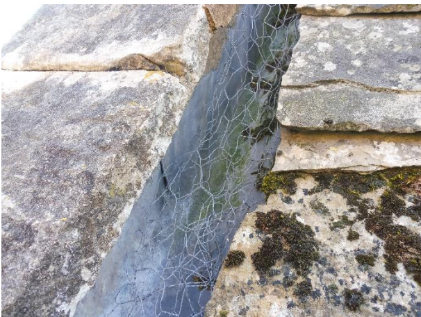
Lady Chapel, north – Wire mesh to lead lined secret gutter.
