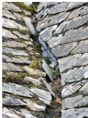
Kitchen/Vestry pitched valley gutter - Significant moss and several slipped slates.
