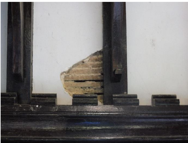
South Porch – Damage to lath and plaster ceiling.
