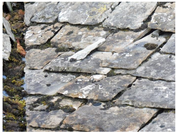
Vestry east – Slipped slates.
