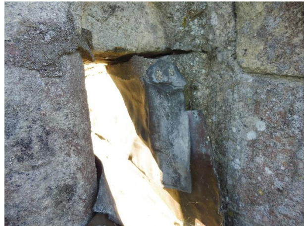
Vestry west lead lined box gutter – Loose and detached cover flashing through outlet.
