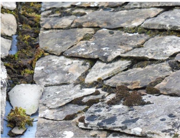
Vestry east – Damaged, slipped and missing slates.
