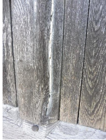
South Porch – Splits/shakes to timberwork filled with dense mortar.
