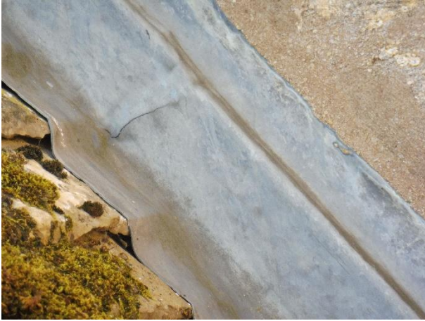
Lady Chapel, north – Split to cover flashing at Tower abutment.
