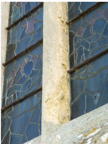
North Aisle – Erosion and minor fractures to mullion and rusting external saddlebars.
