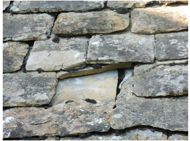
Vestry east – Damaged slate.
