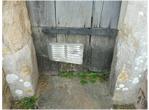
Turret staircase doorway – Splits to boarding and defective vent.
