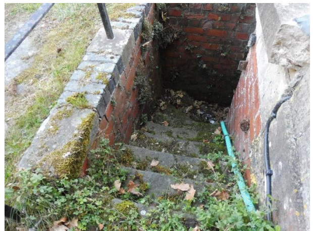
Boiler House steps – Moss and vegetation.
