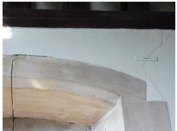
North Aisle – Movement above east window with tell-tale installed.
