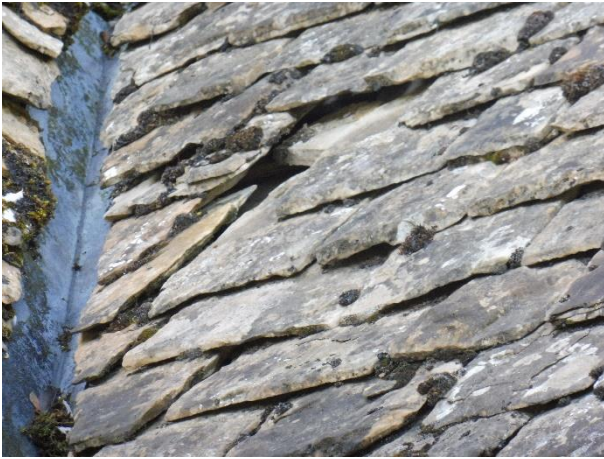
Vestry east – Slipped/missing slates.
