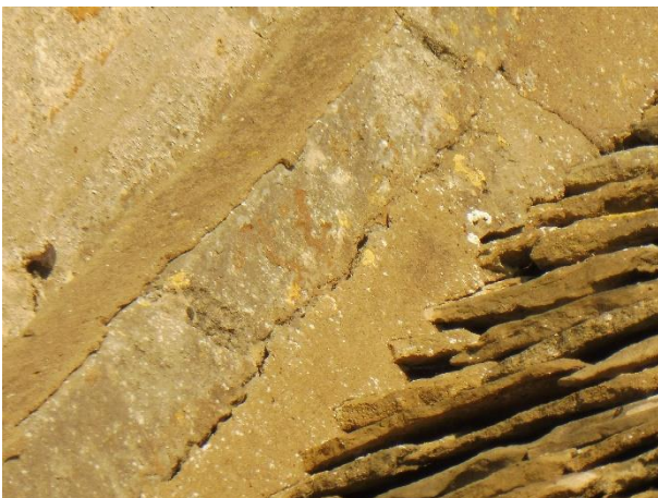
Lady Chapel, south – Cracking to mortar fillet at Tower abutment.
