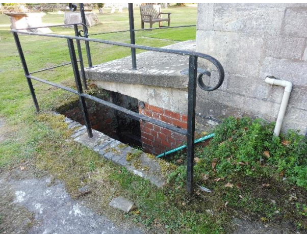
Boiler House steps – No lockable gate.
